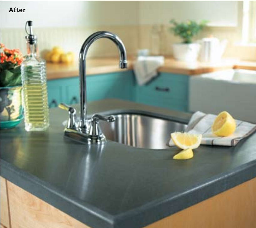
Undermounted sinks have a sleek appearance and make cleanup easy, but they are only a good idea in countertops that have a solid construction, such as solid-surfacing, stone, quartz, or butcher block. Laminate and tile countertops are not compatible with undermount sinks.
