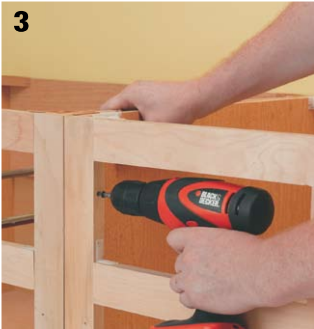
3 Detach individual cabinets by removing screws that hold face frames together.
