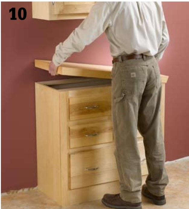
Add the countertop of your choice. See pages 86 to 89 for information on choosing a countertop type and building it yourself. If you are building just a single base cabinet, consider a higher end material such as solid surfacing or granite. The small scale will let you introduce an expensive material without spending a fortune.
