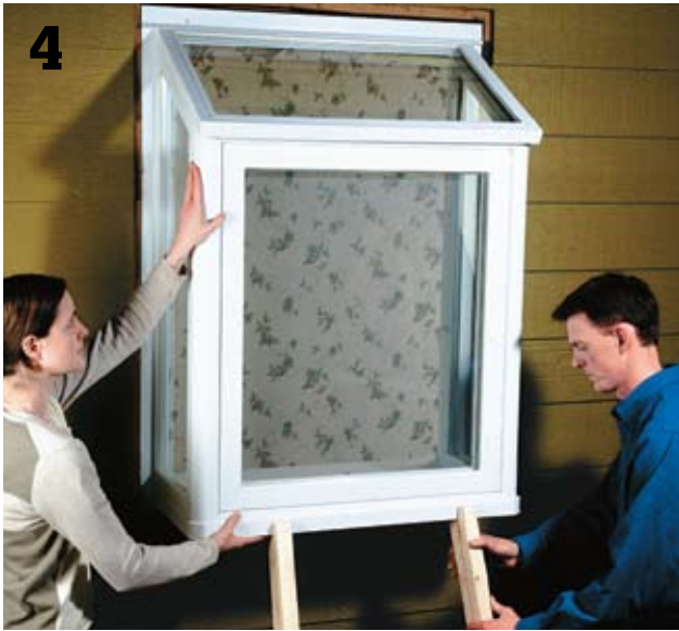
Insert the garden window into the opening, pressing it tight against the framing. Support the unit with notched 2 × 4s under the bottom edge of the window until it has been fastened securely to the framing.
