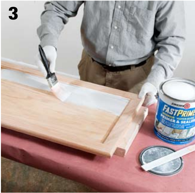
Prime the surfaces. Use a synthetic brush to paint all surfaces with a coat of high-quality, sandable acrylic primer. Allow the primer to dry. Sand with 150-grit sandpaper to remove brush marks and drips.
