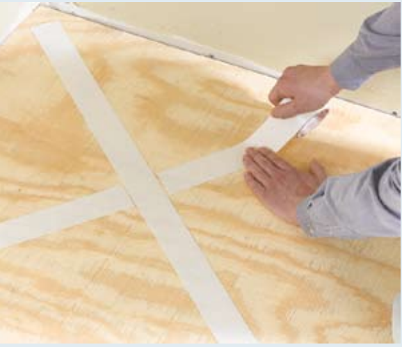
Place acrylic double-face tape in areas that will be under heavy appliances such as stoves and refrigerators. Make an X with three pieces of tape—one long piece and two short pieces—so that the tape does not overlap. Place acrylic double-face tape at doorways and under seam lines. Leave the paper covering in place and press the tape down so it adheres well to the subfloor.
