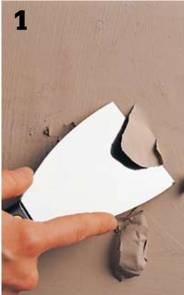
Scrape away loose paint with a putty knife or paint scraper.
