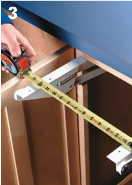
Determine the width of the shelf by measuring between the outer edges of the shelf-mounting flanges.
