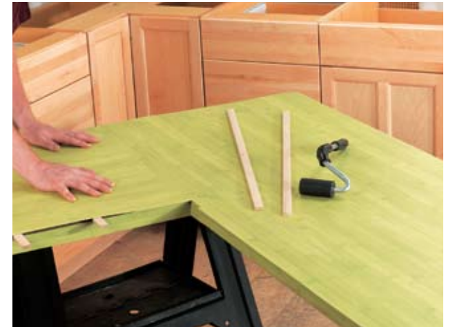
Plastic laminate is bonded to a particleboard subbase with contact cement.
