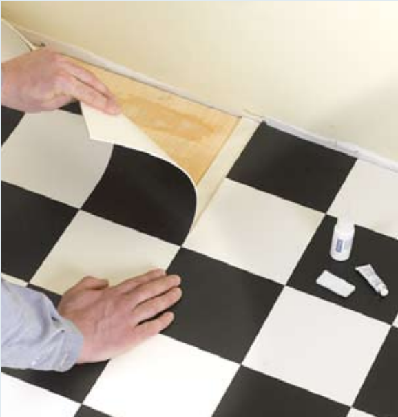
Center the tape under the two sides at seam lines. Press one side of the vinyl into place first. Place the second vinyl sheet and press it into place. Use a seam sealer kit to seal the seams.
