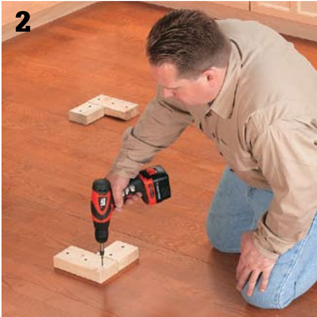
Cut 2 × 4 cleats to fit inside the inner outline to provide nailing surfaces for the cabinets. Attach the cleats to the floor with screws or nails. Tip: Create an L-shaped cleat for each inside corner.
