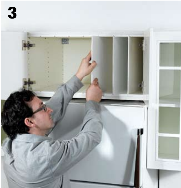
3 Install the top and bottom pieces into the cabinet so the slots are aligned. Fasten the top piece in place with screws. Measure vertically between the slot bottoms, then cut the divider panels 1/16" shorter than this dimension. Slide the panels into place at the desired spacing.
