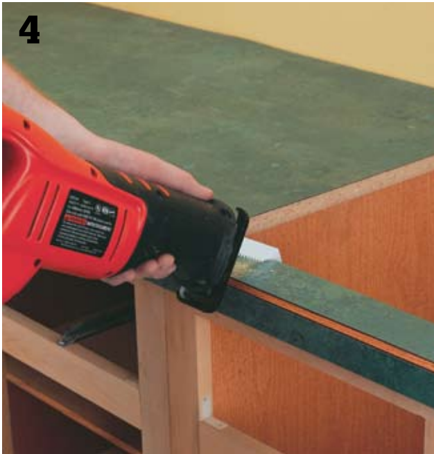
4 Countertops are usually not salvageable. Cut them into manageable pieces with a reciprocating saw, or take them apart, piece by piece, with a hammer and pry bar.
