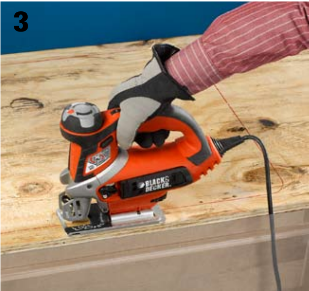
3 Make the sink cutout. To create cutting lines, place the sink upside down in the desired location. Trace the edges of the sink and remove it. To create support for the drop-in sink flange, use a compass to trace new cutting lines inside the traced lines (usually 5/8"). See the manufacturer's instructions to confirm dimensions (some sinks come with a template for making the cutout. Use a jigsaw to cut out the sink opening.
