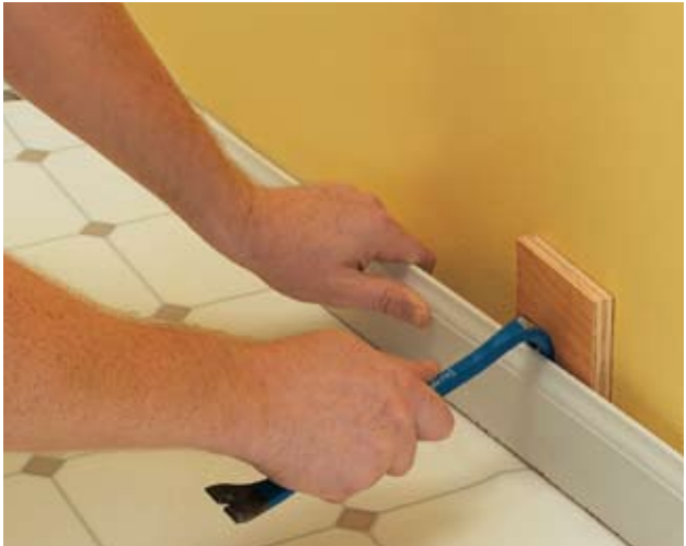
Remove baseboards and other trim moldings with a pry bar. Protect wall surfaces with scraps of wood. Label the trim boards on the back side so you can replace them correctly.
