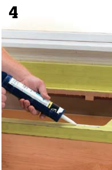
Apply a bead of silicone caulk around the edges of the sink opening. The sink flange most likely is not flat, so apply the caulk in the area that will make contact with the flange.
