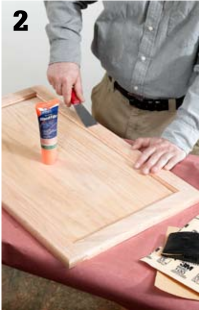
Sand all surfaces with 100-grit sandpaper. Fill all screw holes and nicks and dents with wood filler, and then sand smooth when dry. If you are reusing the same hardware, you do not need to fill the screw holes.
