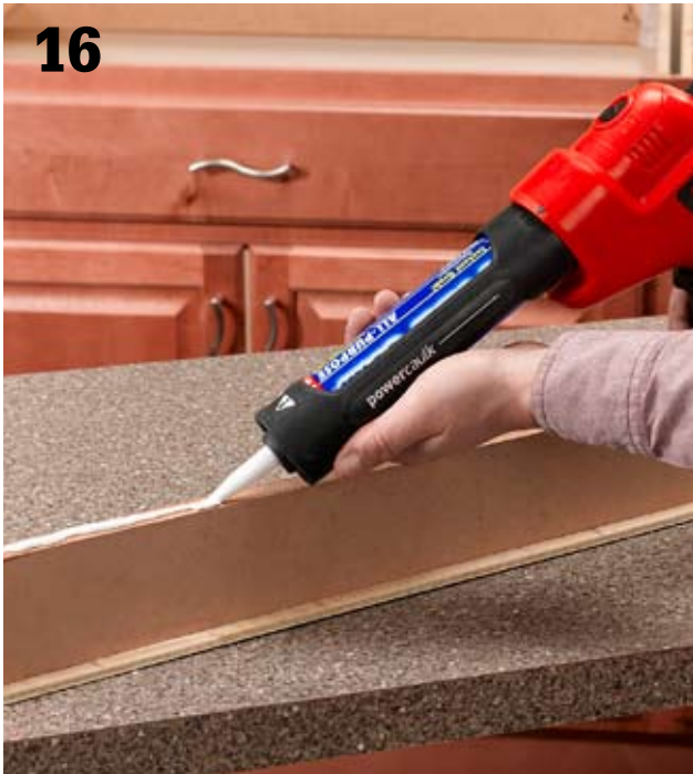
Apply a bead of silicone caulk to the bottom edge of the backplash.
