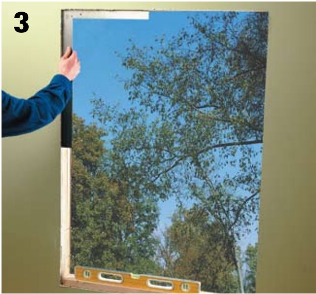
Use a level to check that the sill of the rough opening is level and the side jambs are plumb. Use a framing square to make sure each corner is square. The rough framing must be in good condition in order to support the weight of the garden window. If the framing is severely deteriorated or out of plumb or square, you may need to reframe the rough opening.
