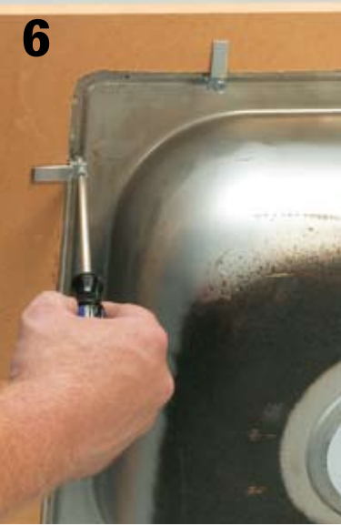
For sinks with mounting clips , tighten the clips from below using a screwdriver or wrench (depending on the type of clip your sink has). There should be at least three clips on every side. Don't overtighten the clips—this can cause the sink flange to flatten or become warped.
