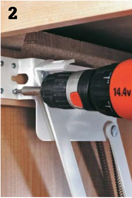
Mark the locations of the swing arm mounting plates onto the inside cabinet faces. Mount a swing arm on each side of the cabinet opening, using screws. Unlock and rotate both swing arms so they are fully extended.
