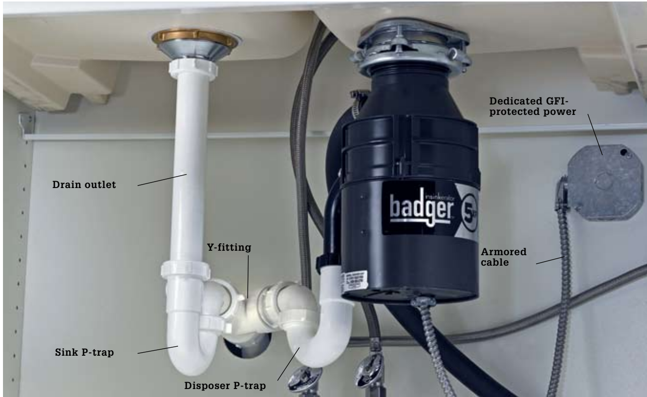
A properly functioning food disposer that's used correctly can actually help reduce clogs by ensuring that large bits of organic matter don't get into the drain system by accident. Many plumbers suggest using separate P-traps for the disposer and the drain outlet tube as shown here.
