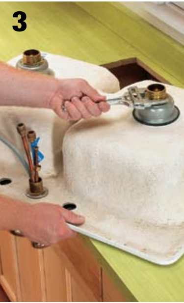
Attach as much of the plumbing as makes sense to install prior to setting the sink into the opening. Having access to the underside of the flange is a great help when it comes to attaching the faucet body, sprayer, and strainer, in particular.
