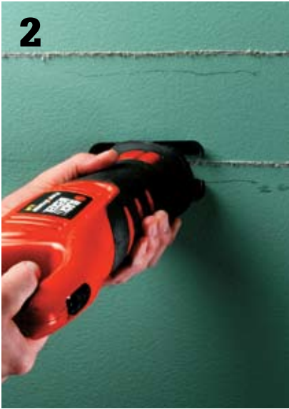
Plan the route for the new supply line beginning at the T-fitting and working toward the cooktop area. Determine the height of the new line and then snap chalklines from the sink to the cooktop. With the electrical power shut off, remove wall coverings 2" above and below the chalkline and at the location for the pot filler outlet. Make sure the location is high enough to clear your tallest stock pot.
