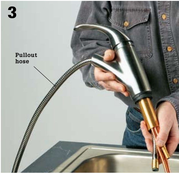
Retract the pullout hose by drawing it out through the faucet body until the fitting at the end of the hose is flush with the bottom of the threaded faucet shank. Insert the shank and the supply tubes down through the top of the deck plate.
