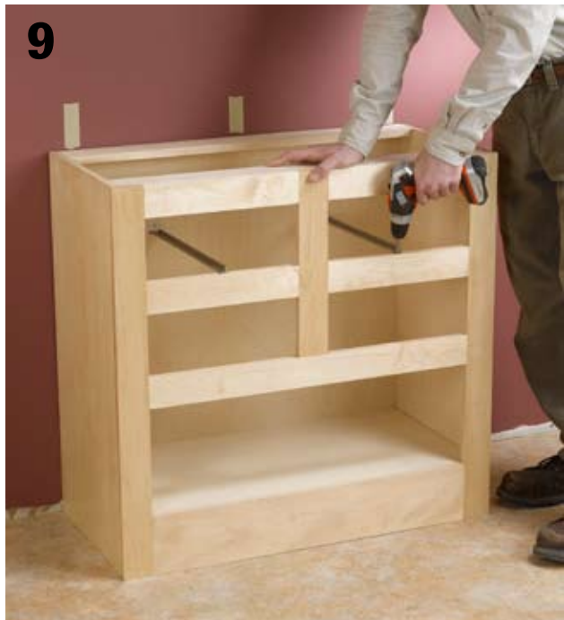
Mount drawer slide hardware in the cabinet interior according to the manufacturer's instructions. Install the drawers and test the fit. Add drawer pull hardware.
