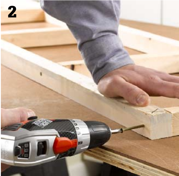
Build a ladderlike framework of 2 × 2s for the soffit sides. If you cannot find straight 2 × 2s, use a table saw to rip 2 × 4s in half. Attach the crossbars at regular intervals of 16" or 24" on center using 2½" screws. Create the ladder so the crossbars will not be aligned with the ceiling joists and wall studs when the framework is installed.
