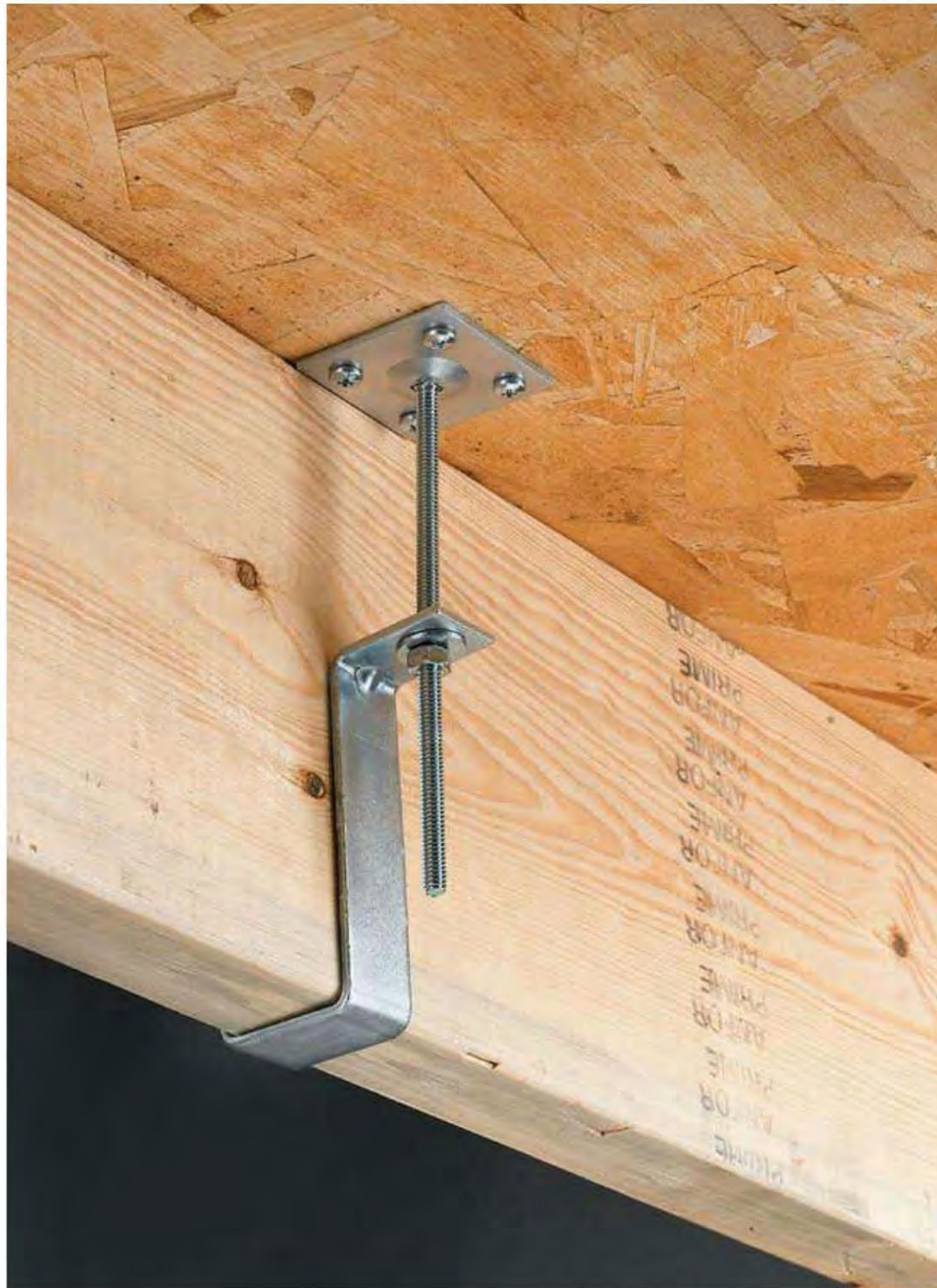
Squeak-elimination tools, such as the Squeak-Ender (shown), tighten the joist to the subfloor and eliminate squeaks. See page 256 for instructions.
