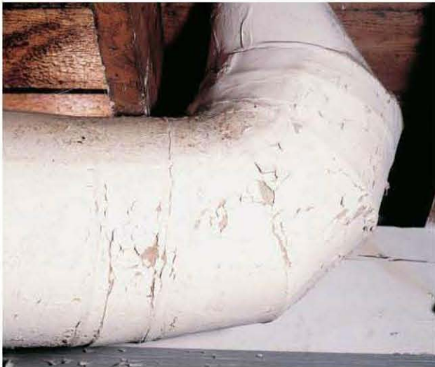
Old insulation containing asbestos poses a serious health risk if it is deteriorating or is disturbed.
