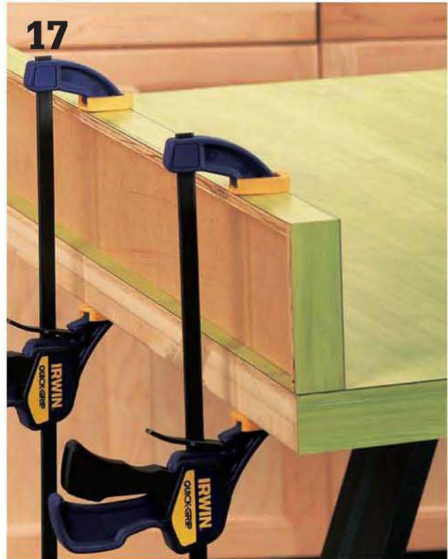
17 Position the backsplash on the countertop, and clamp it into place with bar clamps. Wipe away excess caulk, and let dry completely.
