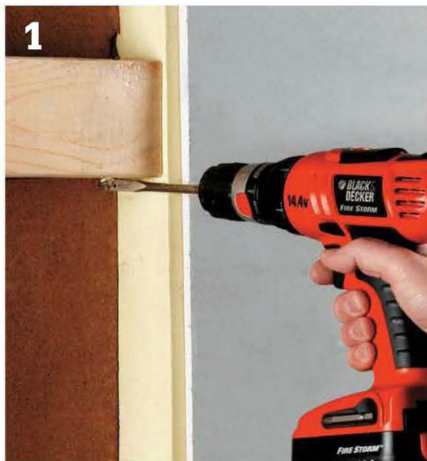
From inside the house, drill through the wall at the corners of the framed opening. Push casing nails through the holes to mark their location. For round-top windows, drill holes around the curved outline (see variation, page 195).
