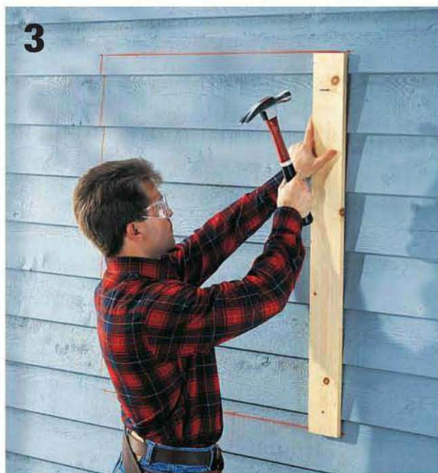
Nail a straight 1 x 4 flush with the inside edge of the right cutting line. Sink the nail heads with a nail set to prevent scratches to the foot of the saw. Set the circular saw to its maximum blade depth.
