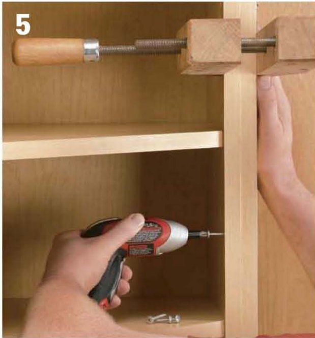
5 Attach the corner cabinet to the adjoining cabinet. From inside corner cabinet, drill pilot holes through face frame. Join cabinets with sheet-metal screws.
