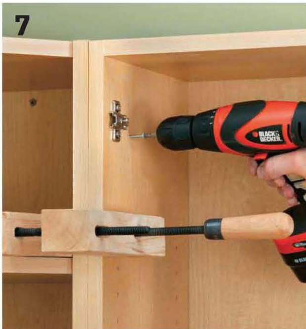
7 Join frameless cabinets with \#8 \times 1\frac{1}{4} " panhead wood screws or wood screws with decorative washers. Each pair of cabinets should be joined by at least four screws.
