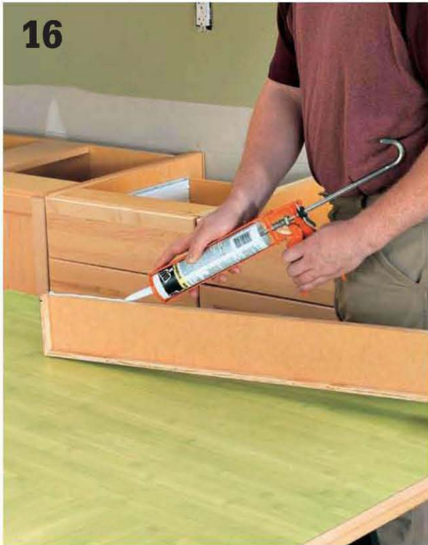
16 Apply a bead of silicone caulk to the bottom edge of the backsplash.
