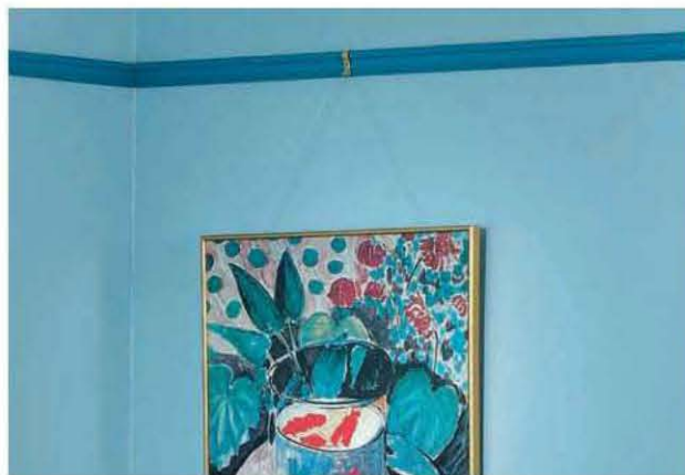
Traditionally, picture rail (see top of photo) is used in conjunction with special hooks to hang artwork in formal rooms without penetrating the wall with fasteners.
