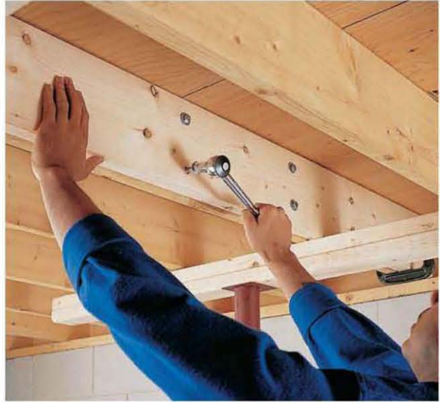
Weakened or undersized joists and other framing members must be reinforced or replaced.
