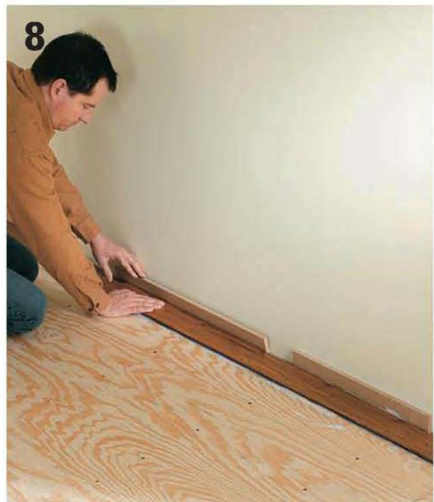
8 Lay the first course of planks with the tongue edge toward the wall. Align the planks with the chalk line. Hold the edge course in place with wedges or by nailing through the tongue edge. This row will anchor the others, so make sure it stays securely in place.
