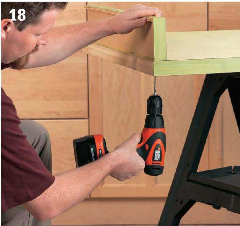
18 Drive 2" wallboard screws through the countertop and into the backsplash core. Make sure screw heads are countersunk completely for a tight fit against the base cabinet. Install countertops.
