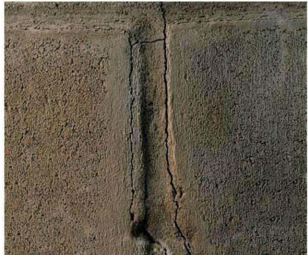
Minor cracks such as these in masonry walls and floors usually can be sealed and forgotten, while severe cracking may indicate serious structural problems.
