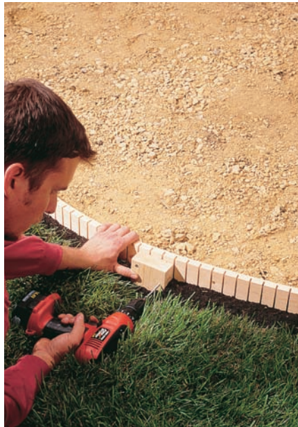
Option: Bend and stake a kerfed 1 × 4 to make forms with curved edges or corners.
