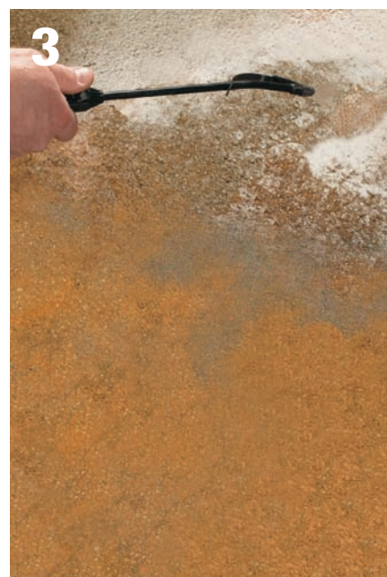
3 Apply a sealer, using a hand-pump sprayer.
