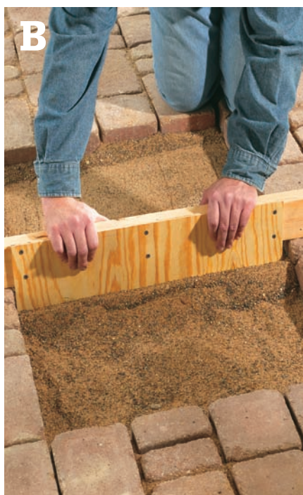
Add or remove sand as needed, then smooth and level the bed using a homemade screed board.
