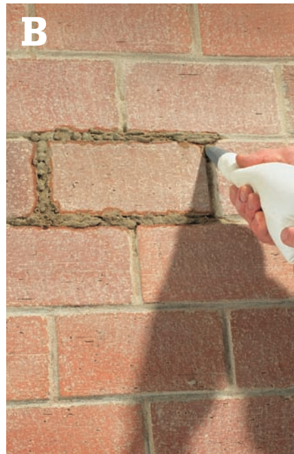
B Use a grout bag or a tuck-pointer to fill the cleaned joints with fresh mortar.
