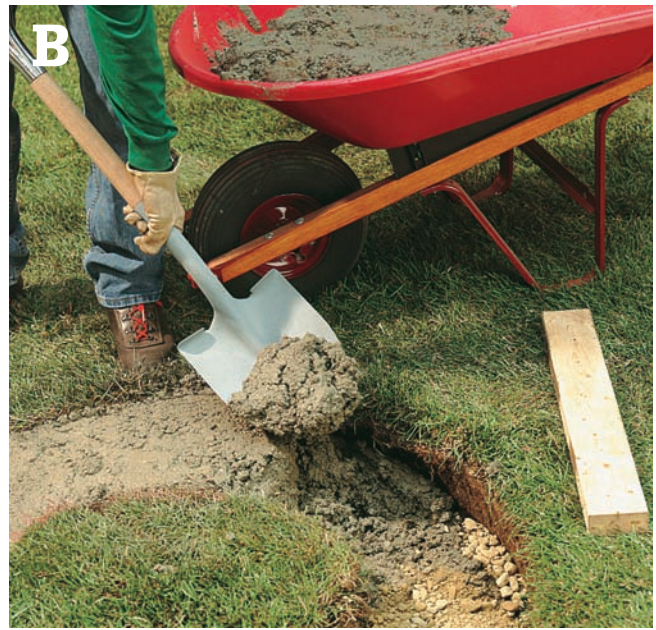
After tamping a 2" layer of compactible gravel in the bottom of the trench, fill with concrete and screed it with a scrap of 2 × 4. Float the surface with a trowel.
