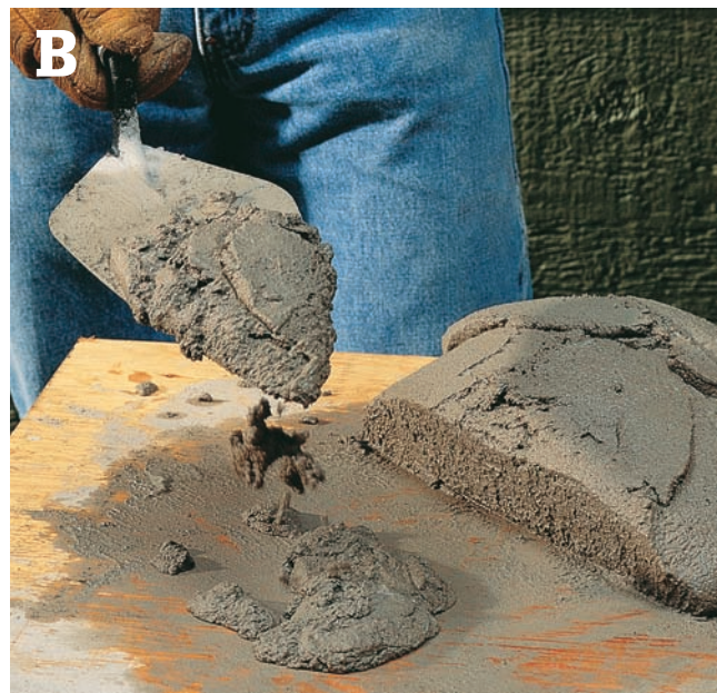
Load the trowel , then snap it down to remove excess mortar.
