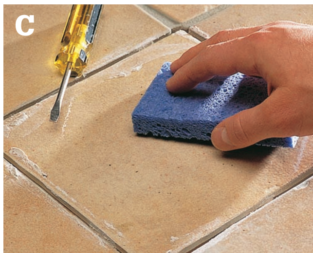
Clean out the grout joints and wipe off the tiles before letting the mortar dry.
