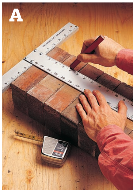
Use a T-square and pencil to mark several bricks for cutting. Make sure the ends of the bricks are aligned.
