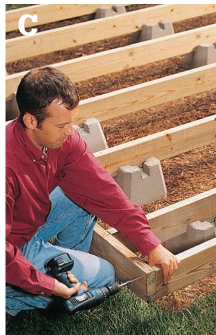
Install the front and back rim joists between the ends of the side joists, securing them with pairs of deck screws.
