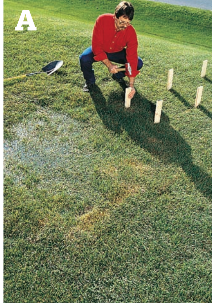
Mark a route for the swale with stakes, making sure that the outlet for the water is at the lowest point.
