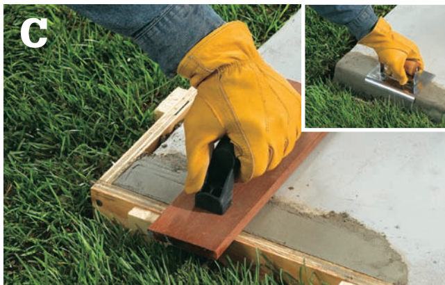
C Smooth the patch with a concrete float. Round-over the top edges of the patch with a concrete edger (inset).
