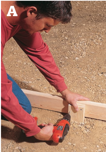
Stake the form every 2 ft. , screwing through the stake to secure the form.
