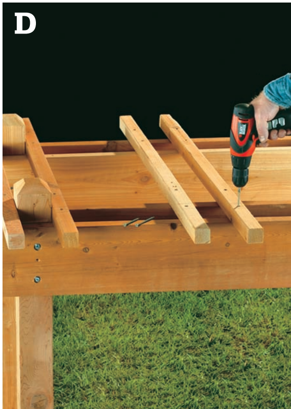
Drill pilot holes for the roof slats, and fasten them to the roof beams with deck screws.
