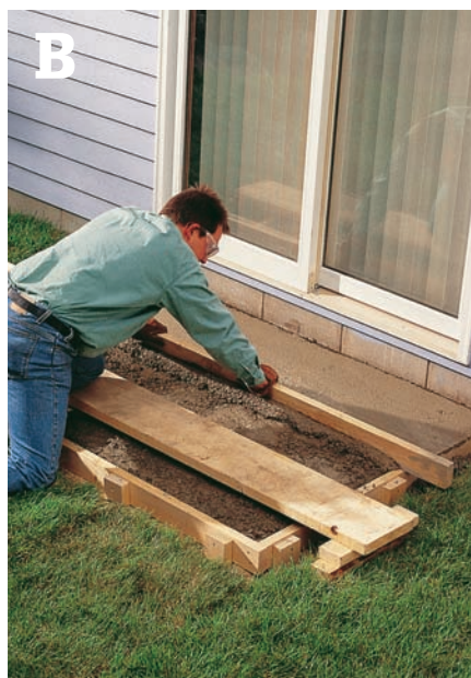
Use a screed board to remove excess concrete before bleed water appears. Use a sawing motion from left to right, keeping the screed flat.
