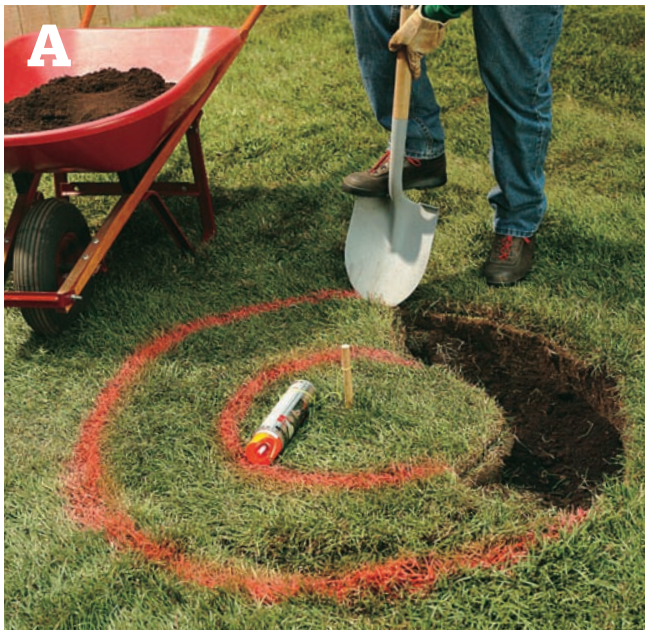
Outline the location of the footing using spray paint and a piece of string. Then dig a circular trench 10" deep.
