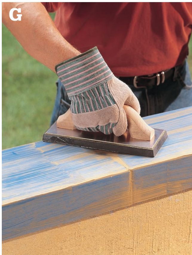
Grout the joints , using a rubber grout float. Wipe the film from the tile and let it dry. Polish the tile with a soft, dry rag.
