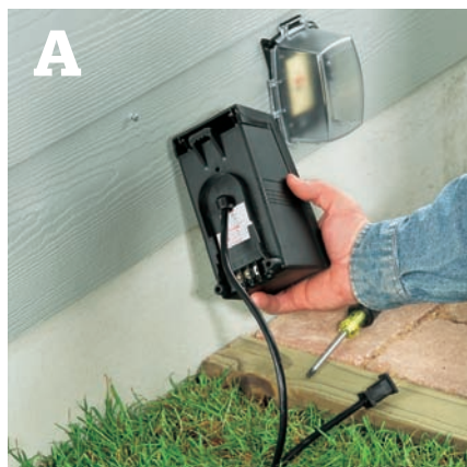
Mount the transformer near a GFCI outlet, following the manufacturer's directions.
