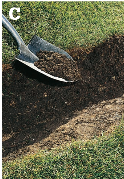
Dig a 6"-deep trench that slopes to the center, creating a V shape. Use the shovel to smooth the sides as you work.
