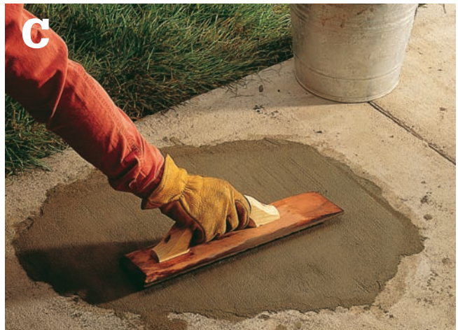
Smooth the patch with a concrete float to blend it into the surrounding surface.
