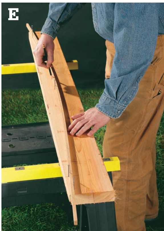
A flexible wood strip helps you make a perfect curve for the long side seat supports.
