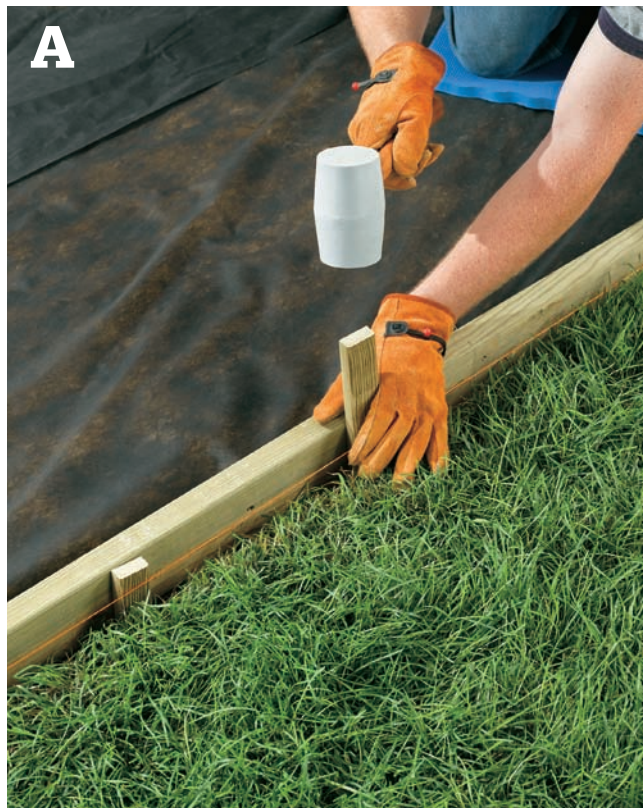
Set the edging boards in place, and then drive stakes below the tops of the boards.
