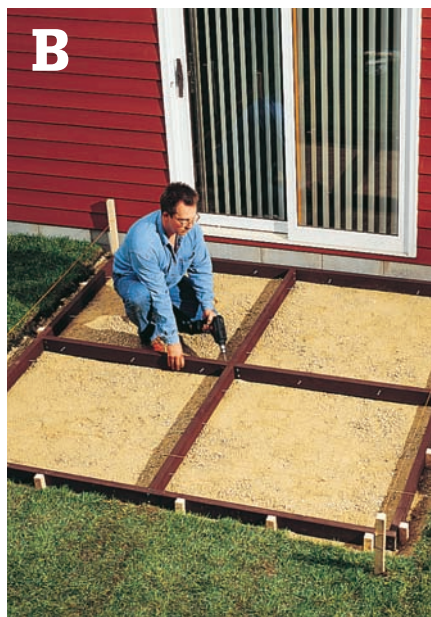
Install dividers between the outer form boards, then add screws for tying the form to the slabs.
