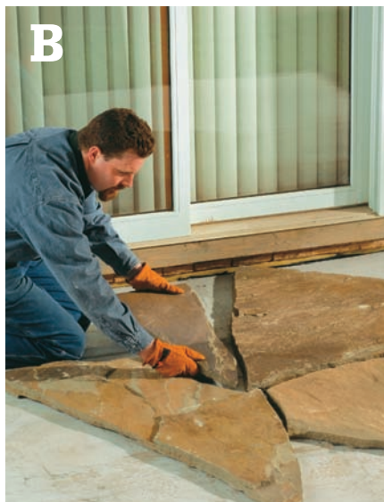
Arrange stones on the patio for an accurate dry-run layout.
