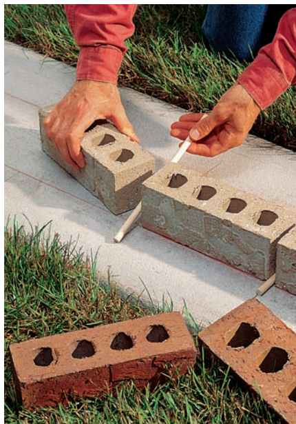
Using wood spacers for mortar joints when dry-laying bricks is a foolproof way to design your brick structure.
