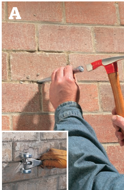
A Chip out the damaged mortar joints, using a small cold chisel. A mortar raking tool is effective for removing mortar close to the surface (inset).
