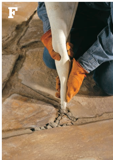
Fill the joints with mortar , using a grout bag for a neat application.
