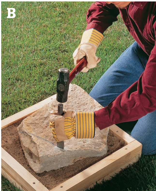
Chisel along the cutting line on the backside of the stone.
