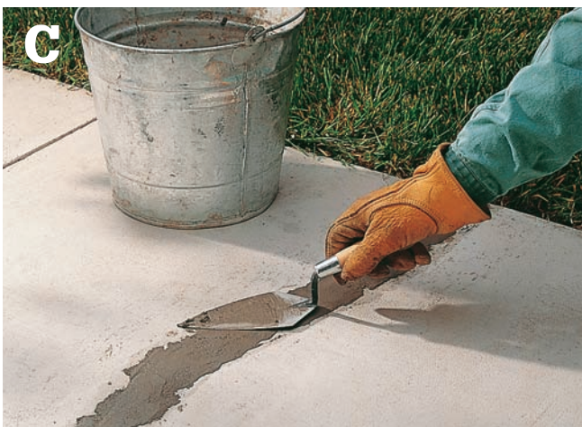
Patch the crack with compound, and smooth the surface with a trowel.
