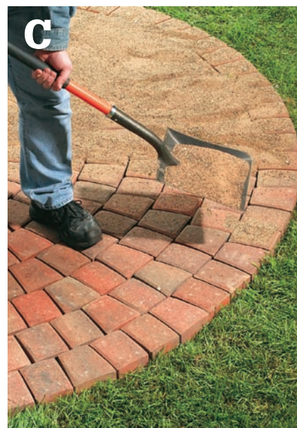
Fill the paver joints with sand, and then pack the surface with a power tamper.
