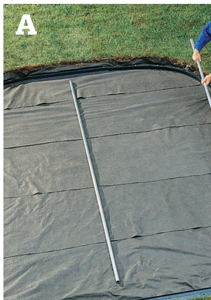
A Lay the screed pipes over the landscape fabric, spacing them to fit the screed board.
