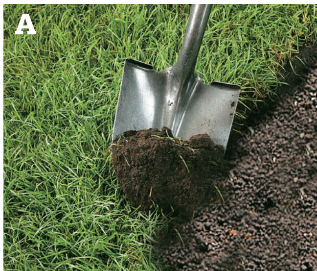
Excavate the site carefully. Dig a trench for edging bricks installed on end.
