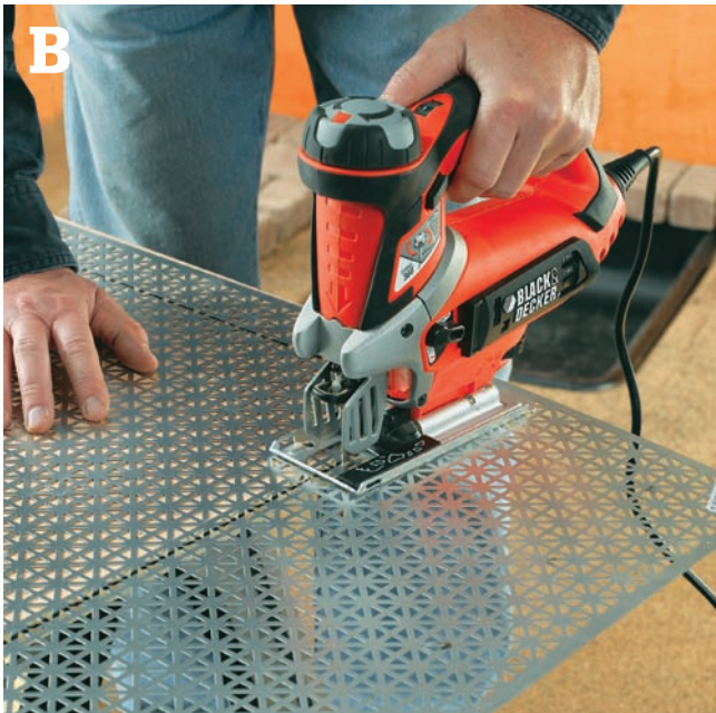
Cut the metal mesh to fit over the top of the reservoir basin, using a jigsaw.
