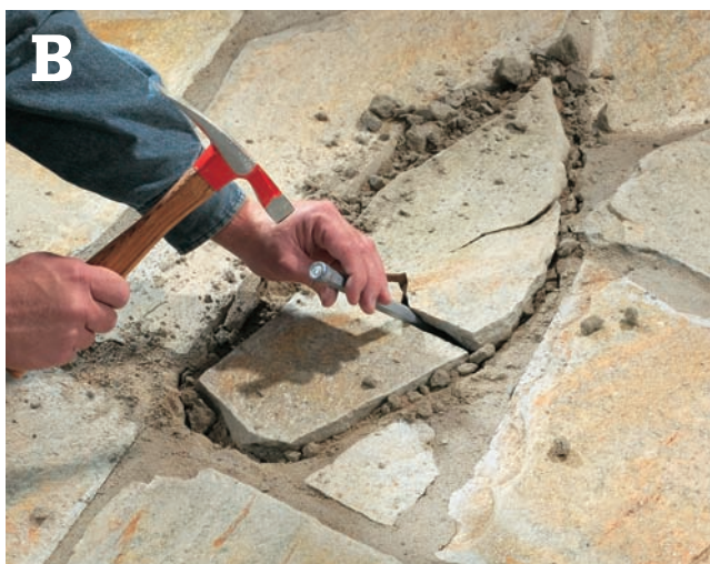
Break up and remove the damaged stone in pieces, then clean out the old mortar bed.
