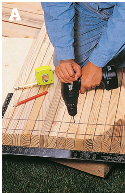
Gang together all of the 2 × 2s, then drill pairs of pilot holes at both ends of each board.
