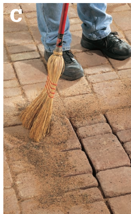
Reset the pavers flush with the patio surface, and then fill the joints with sand.
