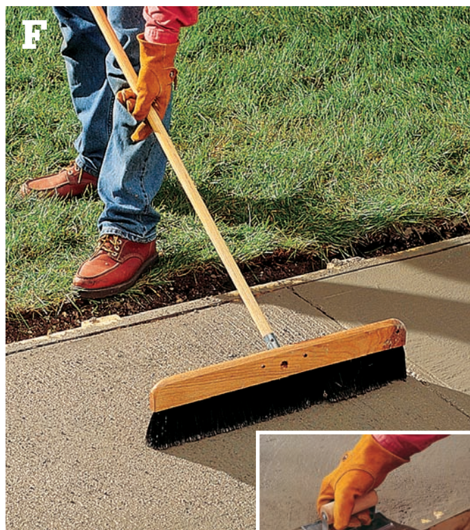
F Shape the edges of the slab with an edger (inset). Broom the surface, if desired, for a nonslip texture.
