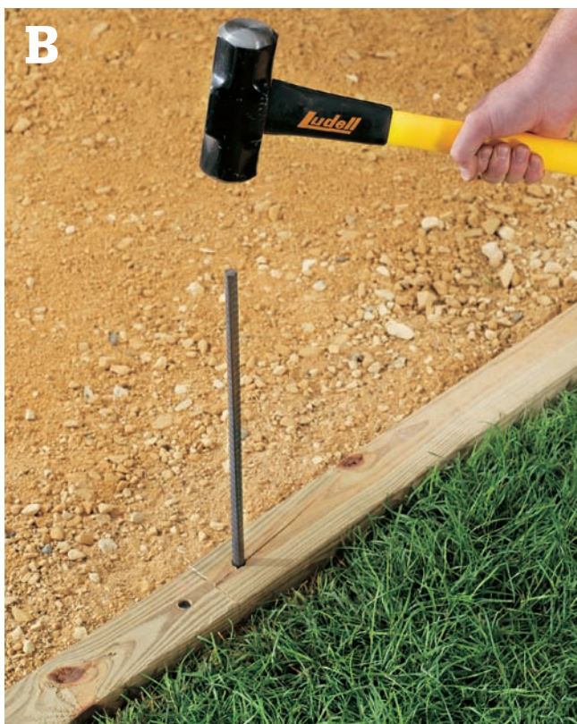
B Anchor the timbers to the ground with 1/2" rebar driven with a maul or sledgehammer.
