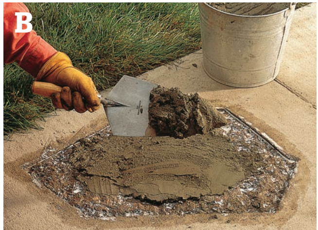
Apply a bonding agent , then fill the area with sand-mix concrete.
