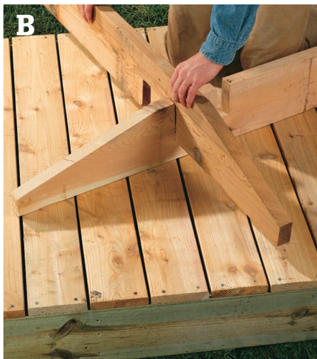
Test-fit the beam joints and make adjustments before installing the beams.
