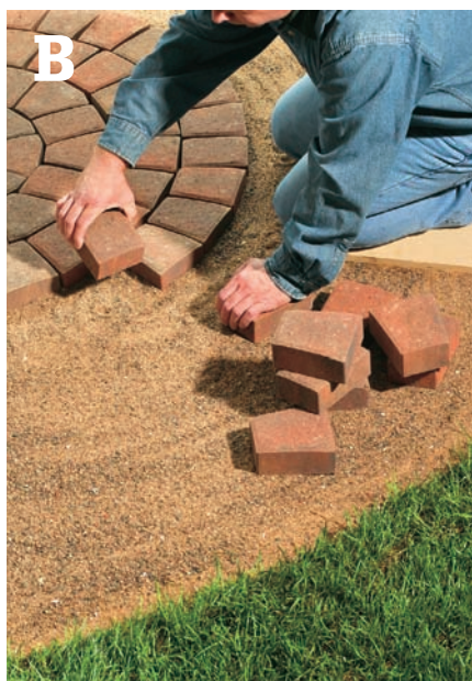
Set the pavers one ring at a time, offsetting the joints between rings.
