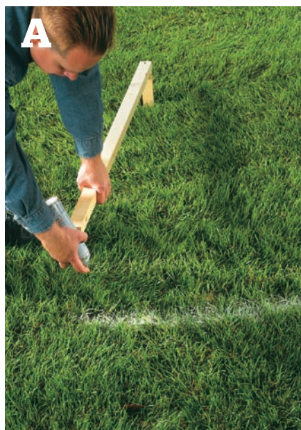
Pivot a board from a central stake to paint the outline of the excavation area.
