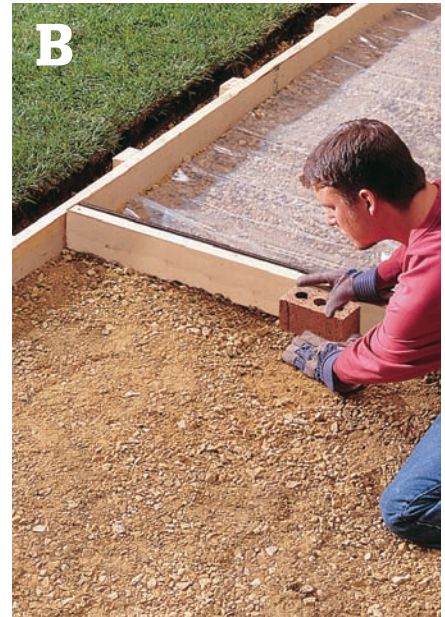
An optional divider separates the slab into workable sections.
