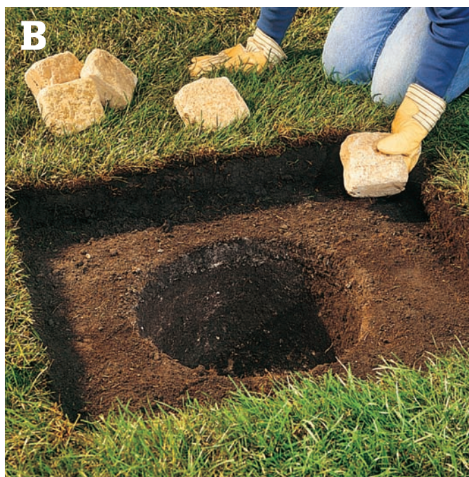
Dig out a 30 x 36" rectangle surrounding the hole, digging 2" deeper than the height of the paving stones.
