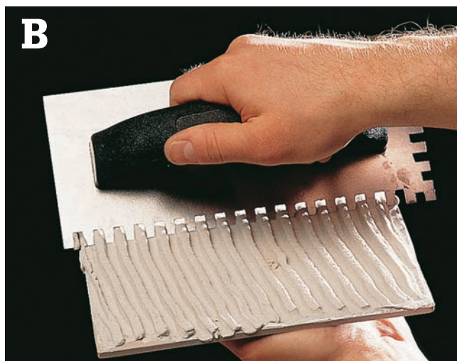
Apply adhesive to the slab surface and the new tile, using a notched trowel.
