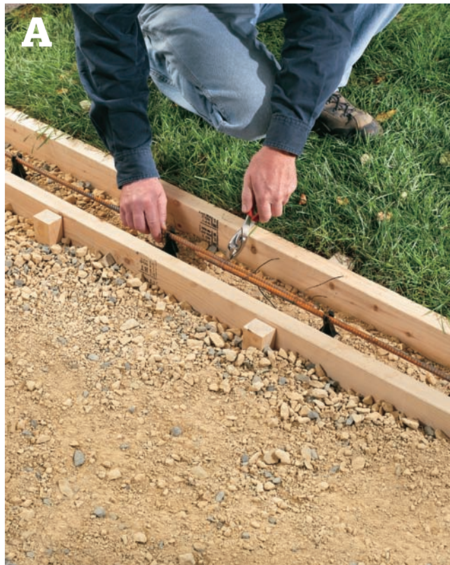
Build wood forms and add rebar to strengthen the curb.
