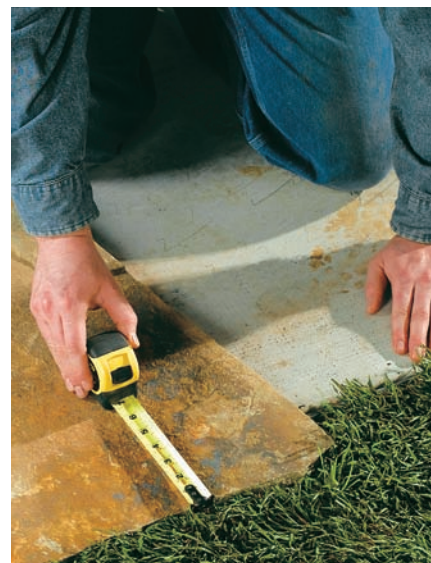
Option: If desired, let outer stones extend beyond the edges of the slab.
