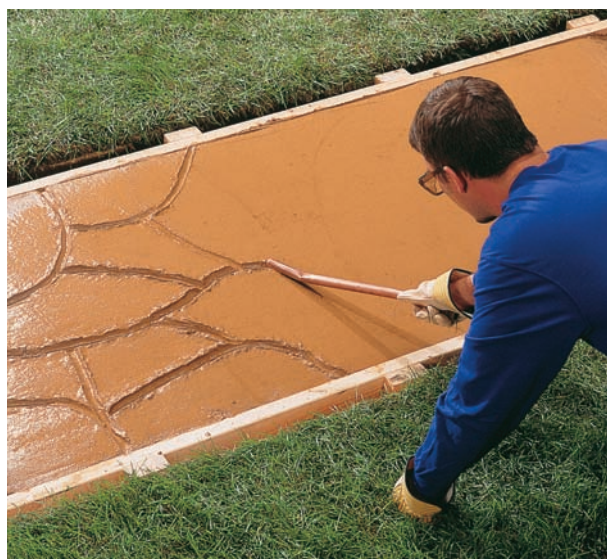
Cut shallow lines in the concrete , using a jointing tool or curved copper pipe.
