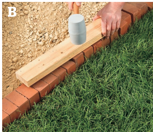
Install edging along layout lines, setting them flush with a mallet and 2 × 4.
