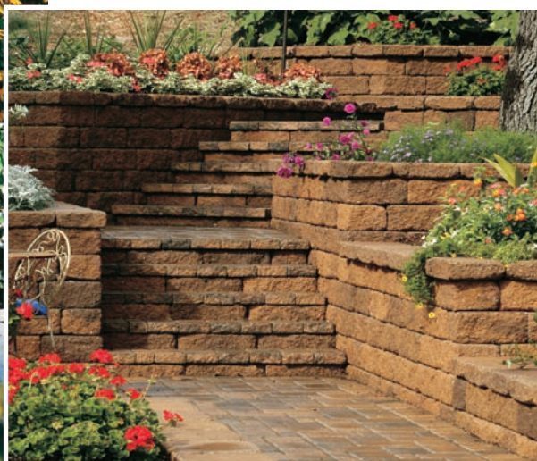
Created with a concrete block system, this patio, stepped walkway, and retaining walls achieve stylistic and structural continuity.
