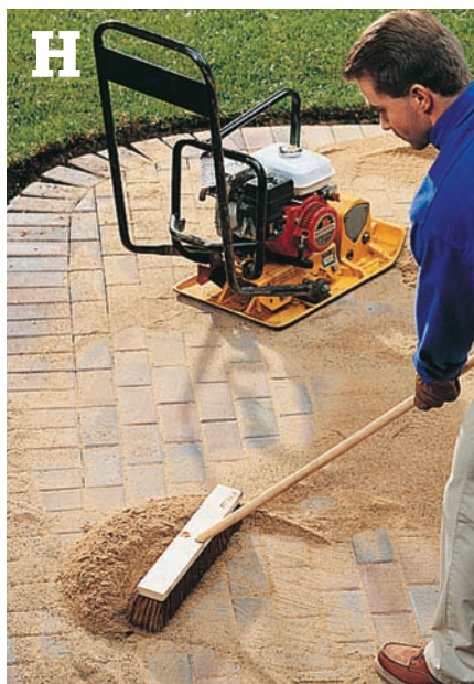
Sweep sand into the joints between bricks, and then tamp the patio with a power tamper.
