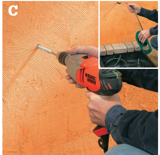
Drill holes for the water supply tube. Use a fish tape to thread tubing inside a framed wall cavity (inset).
