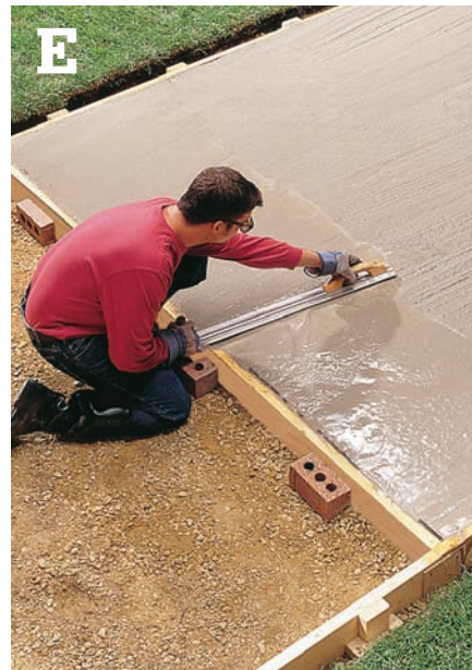
E Let the bleed water disappear, then float the concrete with a darby.
