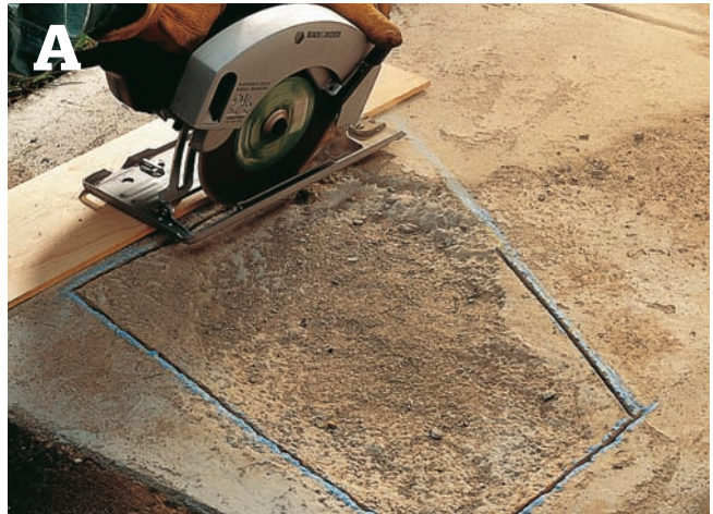
Cut around the damaged area to create a 15° keyed edge for the patch material.
