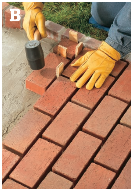
Set the pavers into the mortar bed, using a rubber mallet.
