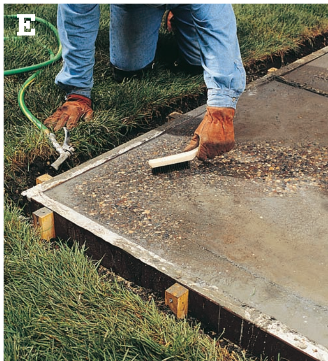
E Scrub the surface with a stiff brush and water to expose the aggregate.
