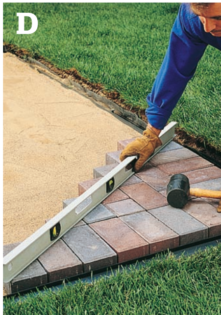
D Check each section of pavers with a level or straightedge to ensure a flat surface.
