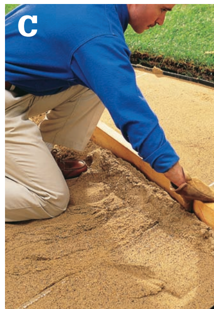
C Pull the screed board along the pipes to screed the sand smooth.
