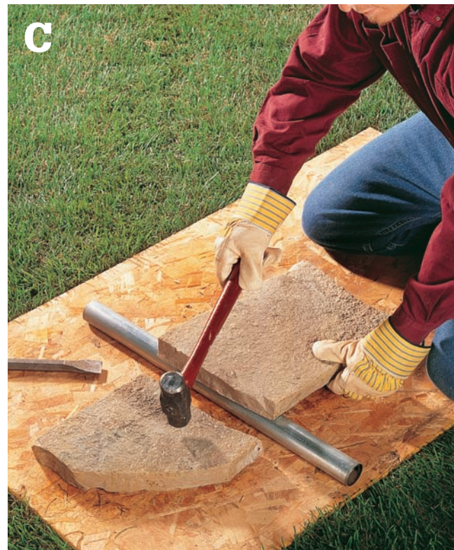
Place a pipe under the cutting line, then strike the waste end to break the stone.
