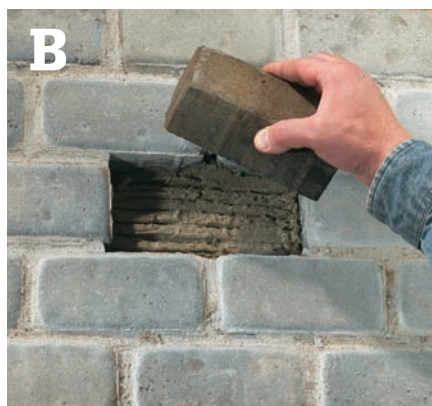
Set the new paver into the mortar so it is flush with the tops of the surrounding pavers.
