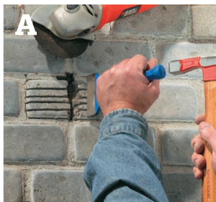
Carefully break out the paver and surrounding mortar, using masonry chisels.
