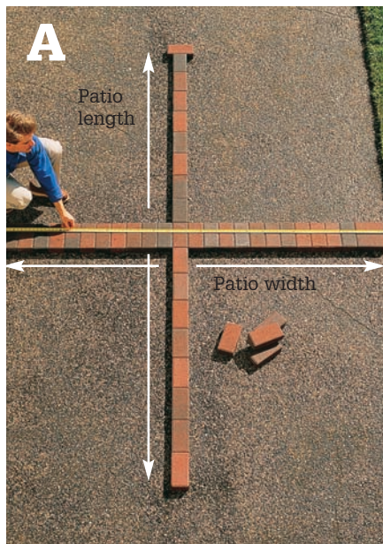
Dry-lay rows of pavers to find the dimensions of the patio surface.
