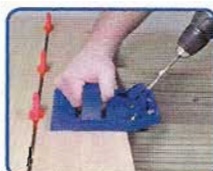
Drill holes into the edge of the deck board using the specialized step bit and the Deck Jig's steel drill guides
