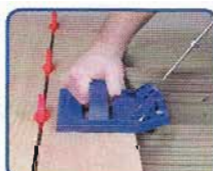
Drive screws through the same drill guide and into the joist while the depth collar precisely controls your depth
