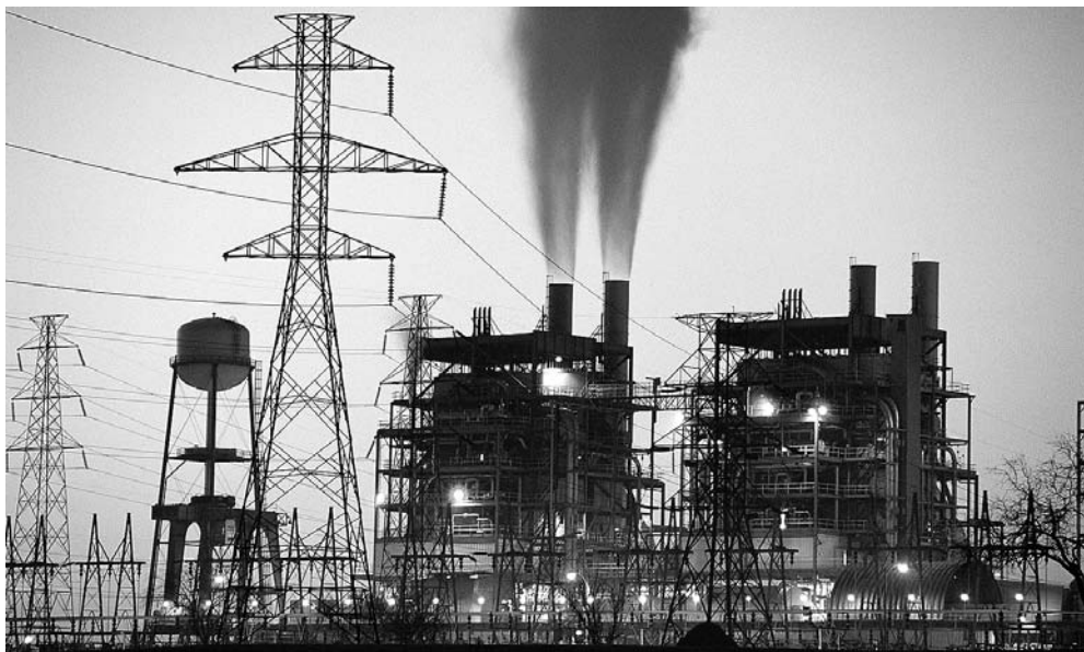
The electricity we use is made by huge machines, or generators, in power plants like this one.
