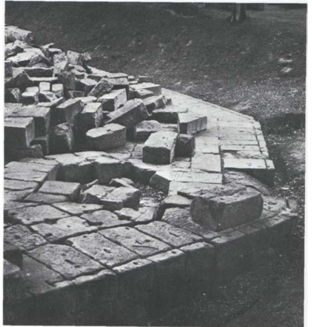
The bridge abutment at Chesters, where the Wall crosses the North Tyne; in some of the stone blocks 'Lewis holes' are still clearly visible.
